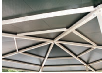
INSULATED SANDWICH PANEL 3" THICK X 48" WIDE, HIGH DENSITY POLYSTYRENE BETWEEN TWO LAYERS OF STUCCO EMBOSSED .032 ALUMINUM
