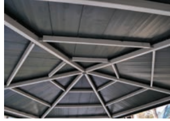
18" WIDE STANDING SEAM PANEL • GALVALUME STEEL, ASTM A792 GR 50
