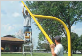
Tip Crossbar to Level and Clamp
