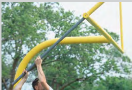
Rotate Upright to Vertical
