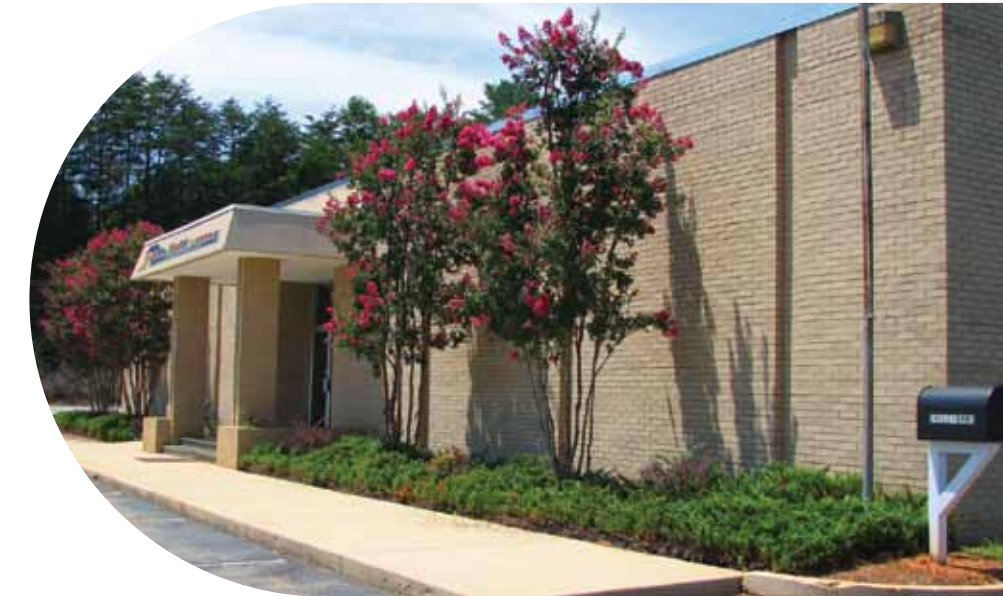
OPERATIONS FACILITY, LENOIR, NC
