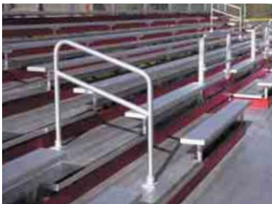
Aisle with Handrail
