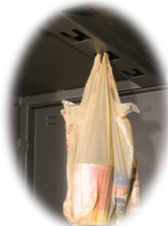
Hooks cut into top support channel inside the locker hold bags for access and organizing supplies.
